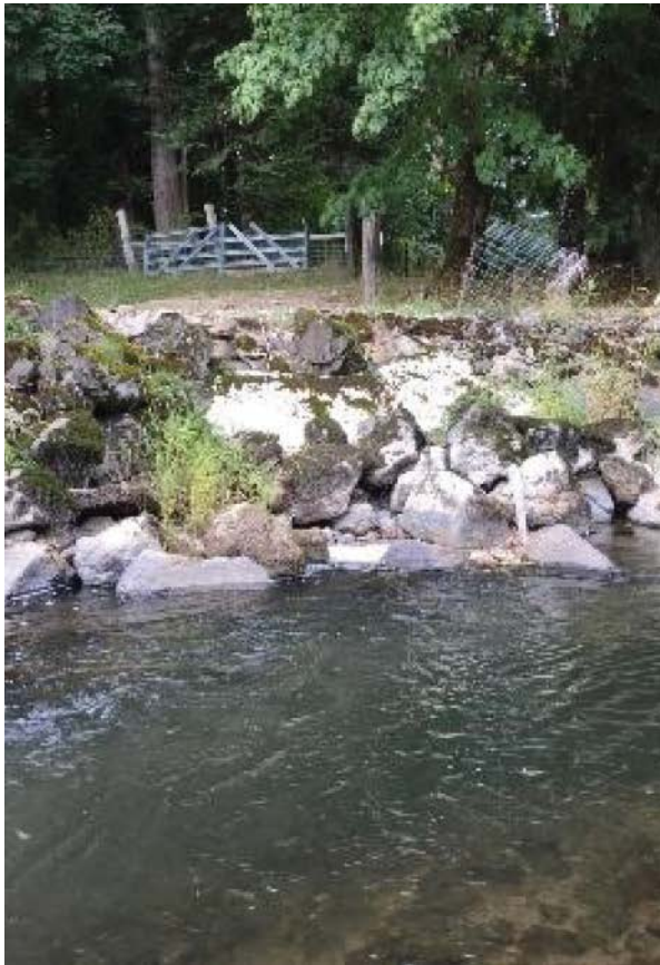
Figure 20. Examples of South and North Fork Newaukum River bank armoring that results in loss of cover and shade, as well as limiting floodplain formation and wood recruitment which is essential to sustaining salmon habitat.
